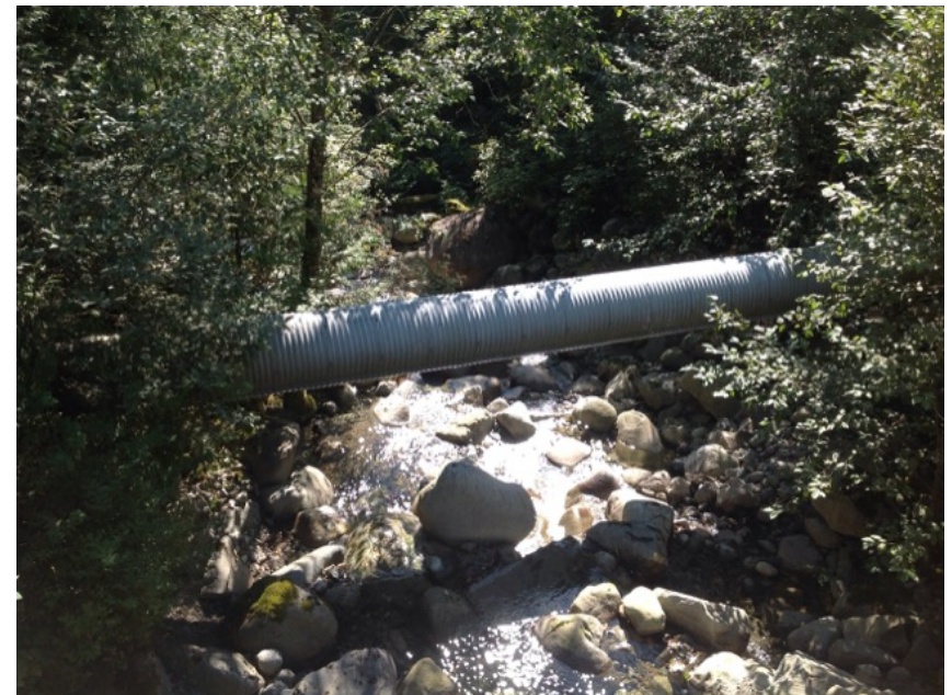
looking downstream from deck
