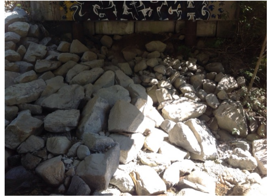
Left Bank Abutment when facing downstream
