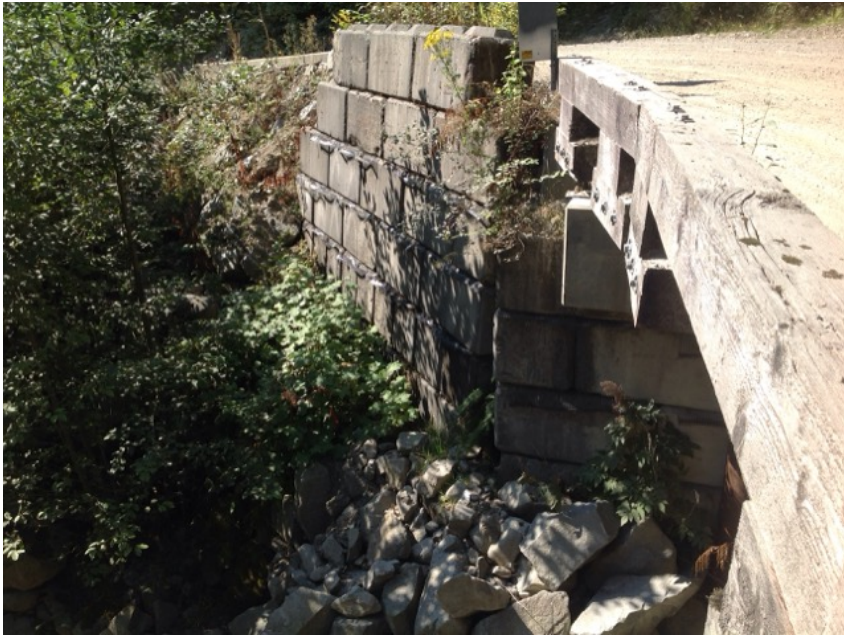
downstream right bank wing wall
