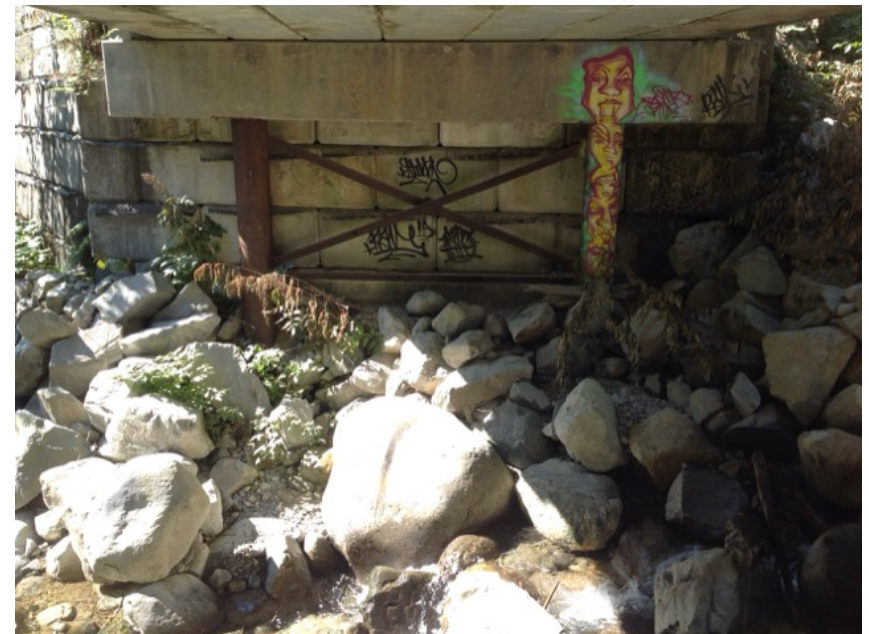
Right Bank Abutment when facing downstream
