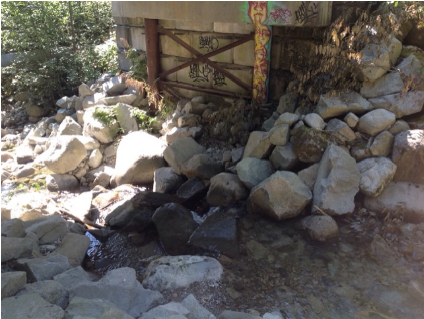
Right Bank Abutment when facing downstream
